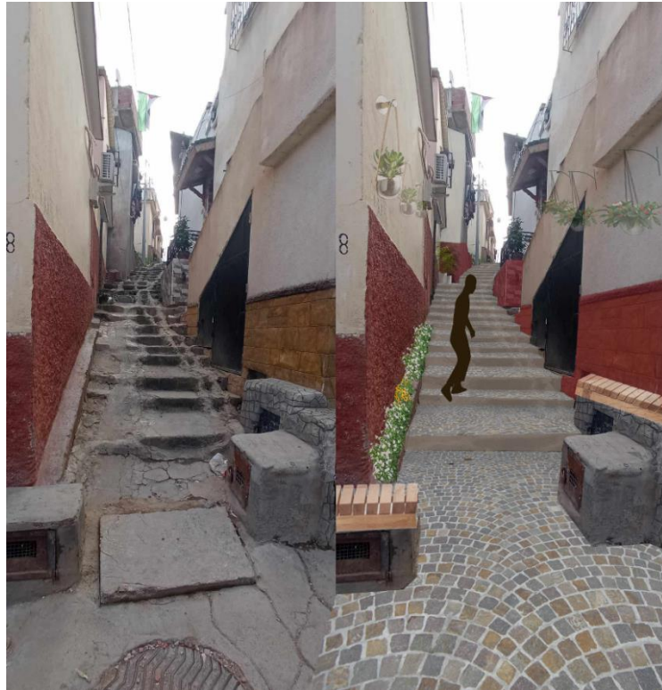
the before and after of the local stairs in Douirette, source author
