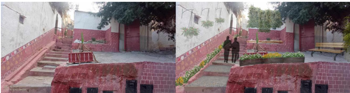
the before and after of the local stairs in Douirette, source author
