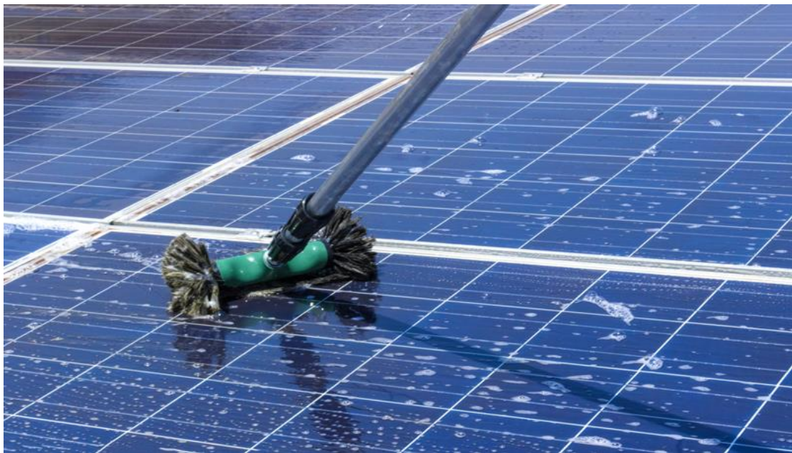
Figure 9: Cleaning solar panels using water [30].
