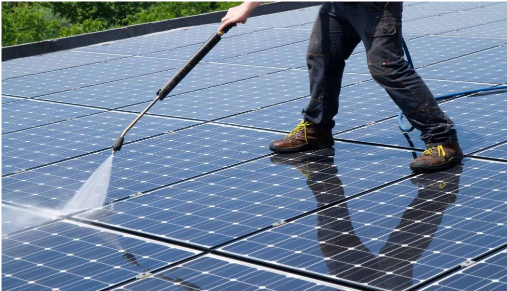
Figure 20: Manual cleaning using water-fed pole.[51]
