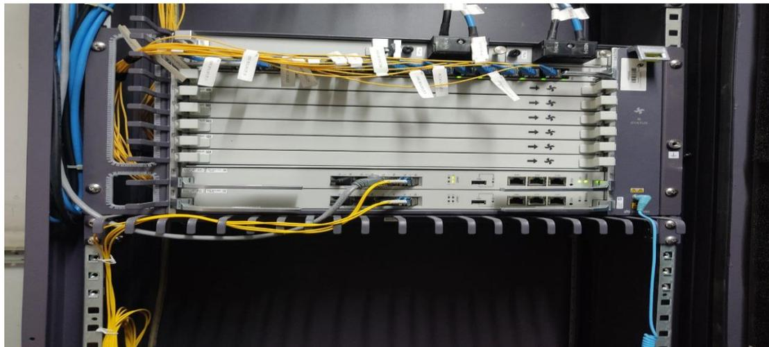
**Figure 2. 6:** OLT (Optical Line Terminal)
