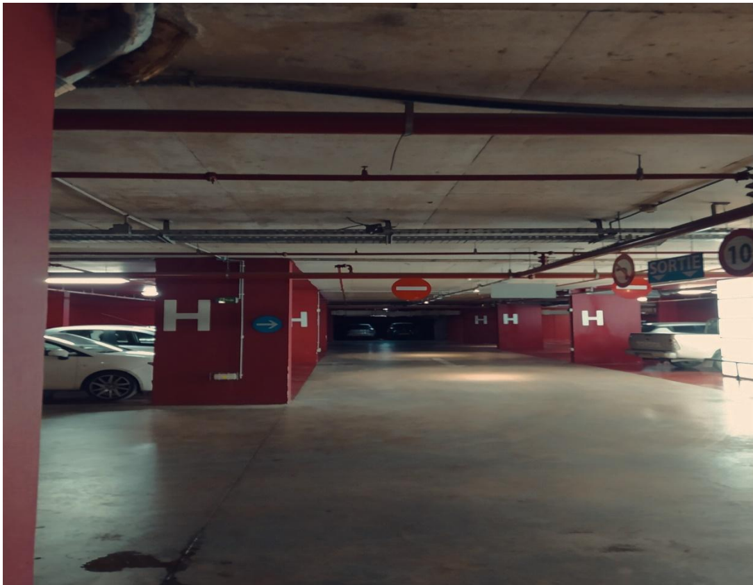
Figure II. 27 Parking de centre commercial garden city
