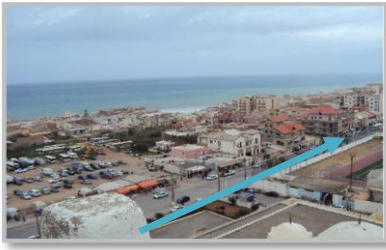
Fig.2.81 Le boulevard Sidi Mhamed
