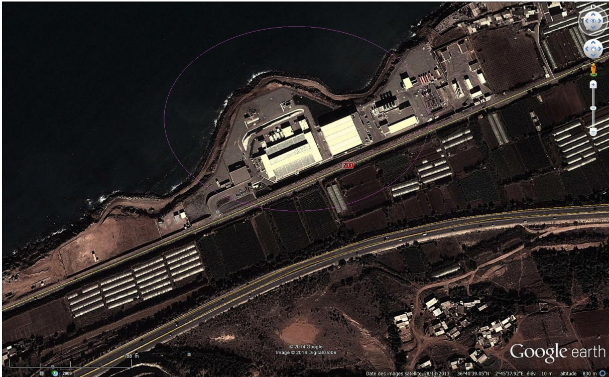
Figure V-1 : Photo de la station de Fouka, [source: google earth]
