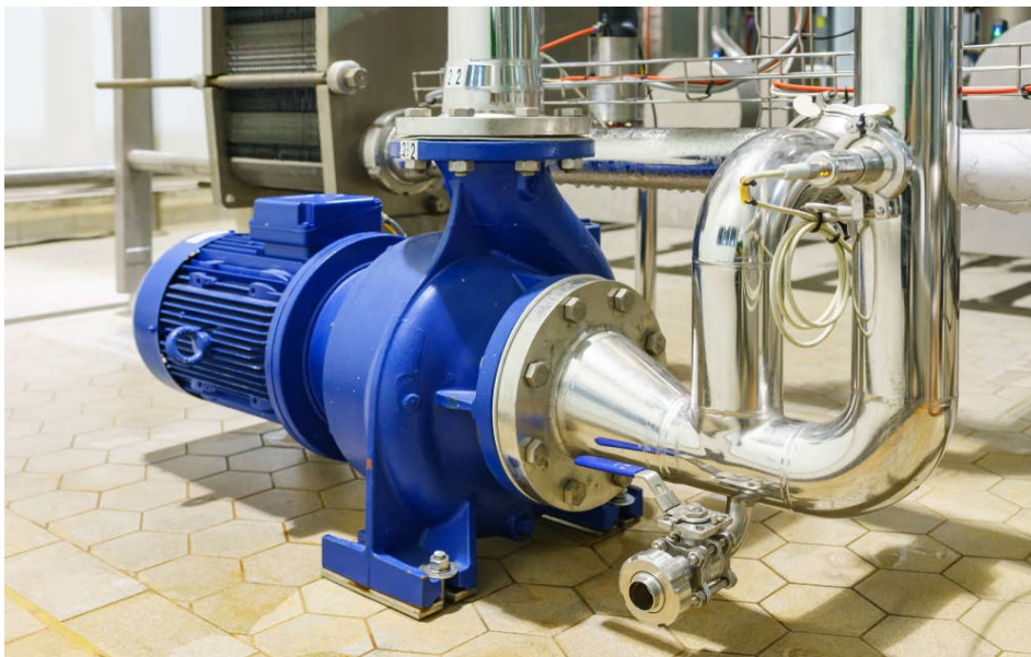
Figure IX.1: pompe centrifuge
