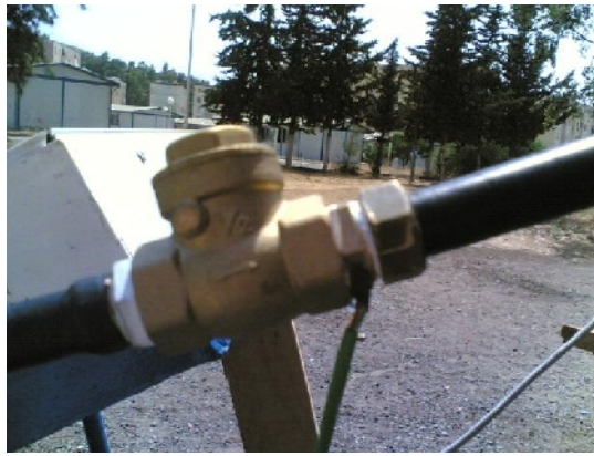
Figure (4-5) : clapet anti-retour
