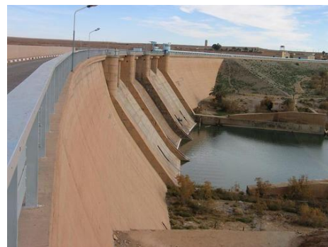
Figure 15: Barrage Dorf Torba
