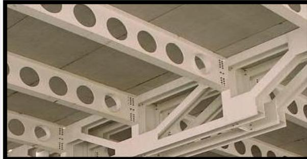
FIGURE 75: POUTRES ALVEOLES, SOURCE ;W
