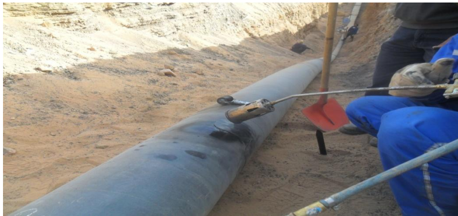
Figure 3.41 : Application de PERP
