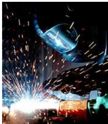
Figure ( II-35) Application de la soudure
