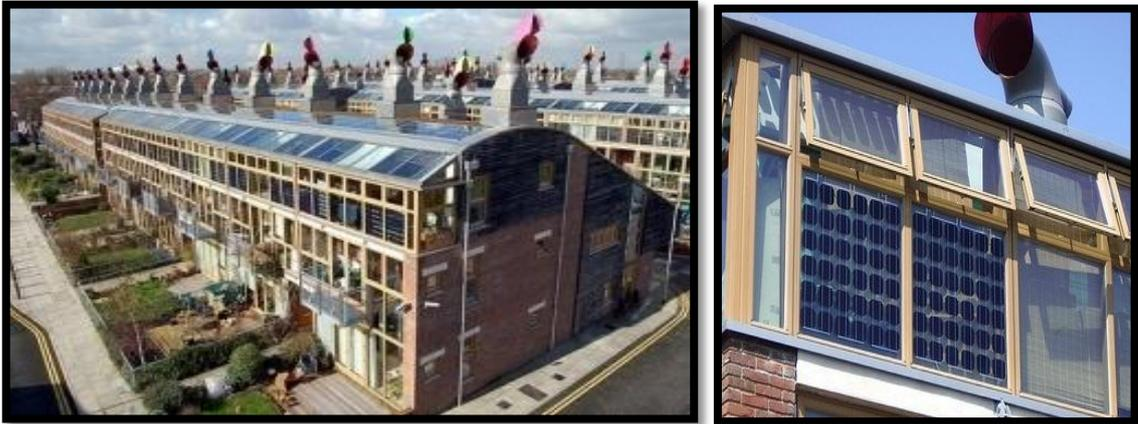
Figure II-24: Panneaux photovoltaïques
