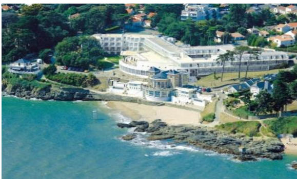
Figure 60: L'hôtel Alliance Thalasso & SPA Pornic/ France
