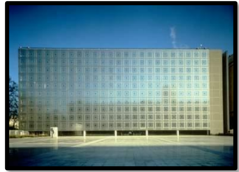
Fig 89. Institut du monde arabe Source: http://www.greatbuildings.com/buildings/L_Institut_du_Monde_Arabe.html
