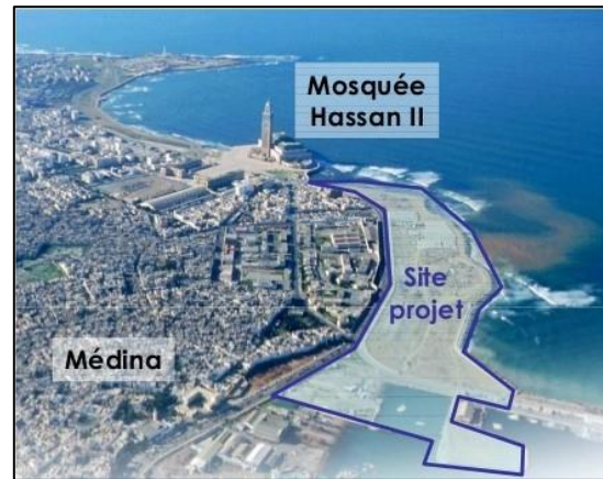
Fig (02) 07 : Situation de Casa Marina. Src : https://Archimag-mag .
