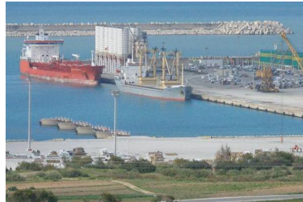
Figure33: Port de DjenDjen, Djijel
