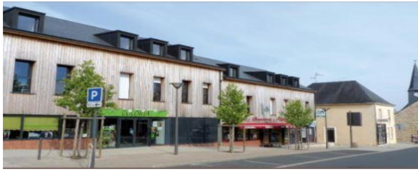
Figure 6: Renouvellement urbain et densification , la Milesse (source: https://www.caue44.com/IMG/pdf/ECOQUARTIER_urcaue_.pdf )
