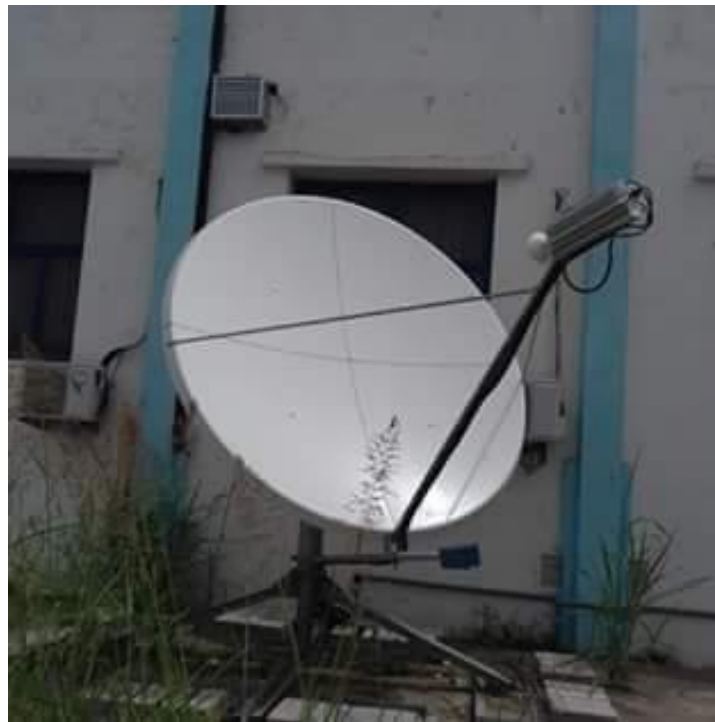
Figure II.15: Antenne VSAT
