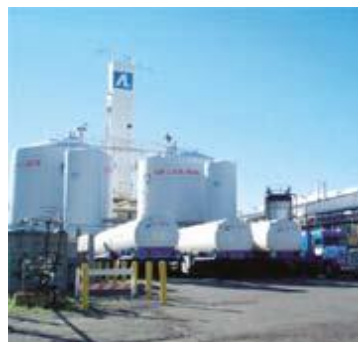
Figure 1.2 : Usine de vaporeformage [27]
