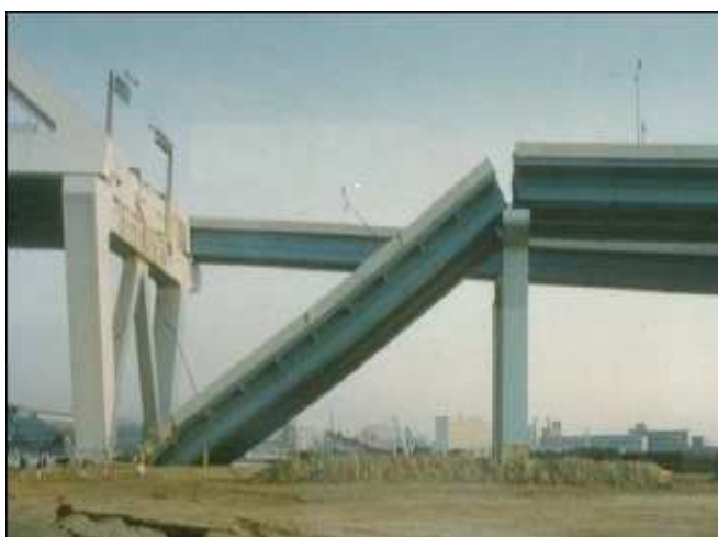
Figure 2.2: Echappement longitudinal (Kobé,1995) [22].
