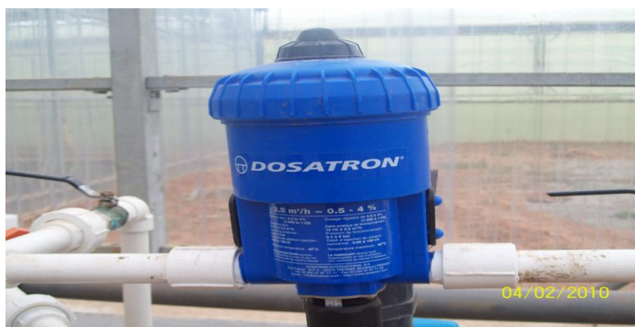
Figure 4.9: Pompe doseuse type Dosatron (Originale, 2010).
