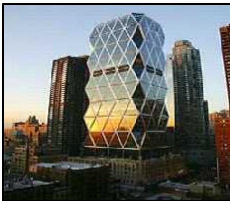
Figure II. 52 : Hearst Tower ; New York. (Source: site web:filtersfast)
