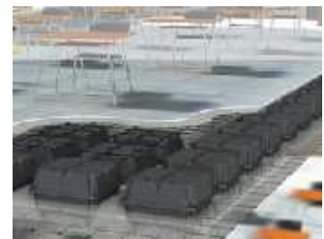
Figure 79: plancher U-boot Source : Kortebj.T,(2017),Technologie U-boot béton
