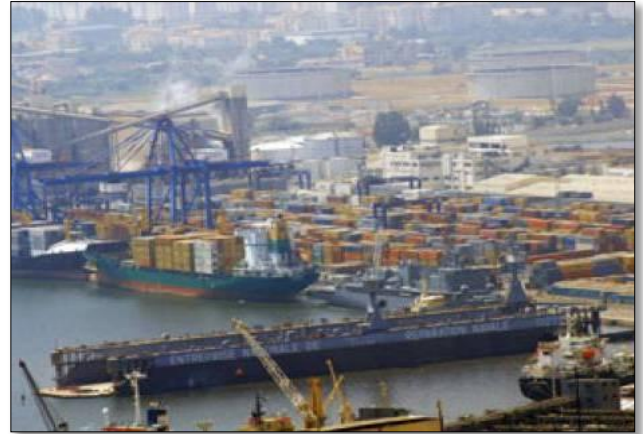
Figure 2: Le port industriel de Bejaia Source: www.portindustriel.com .
