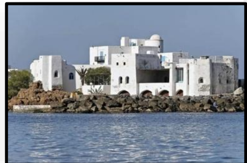
Figure 3:CET Source: www.ComplexeCET.com
