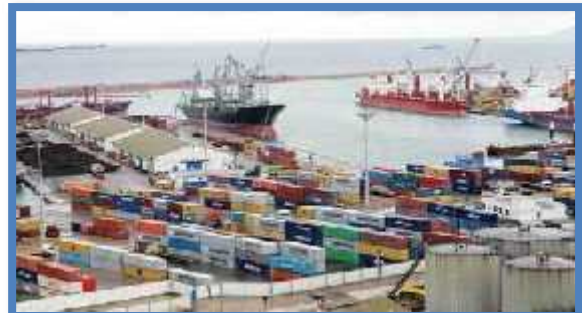
Fig 14: Port industriel d'Alger Source: http://www.lepointeco.com
