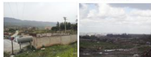
La station de relevage
