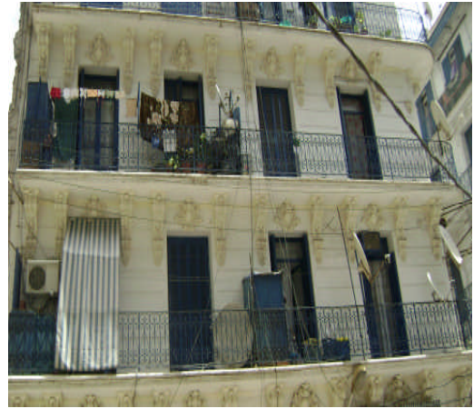
Figure 3.11 : façade principale B
