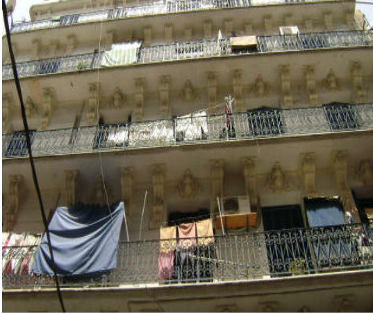
Figure 3.10 : façade principale A
