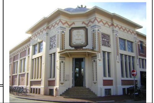
figure I.2.3.33: Bègles - La piscine.
