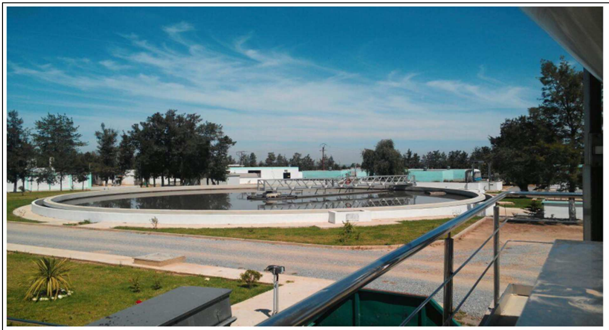
Figure 04. Photo de la station d'épuration de Beni-Mered
