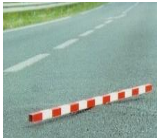
Figure 1.26 : Bourrelet transversal [11].
