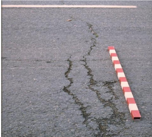
Figure 1.27 : Fissures transversales [11].
