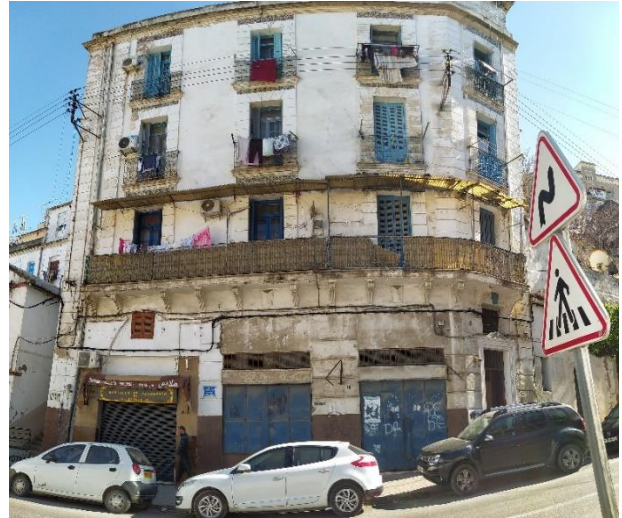
Figure 42 Façade 2 plot 3 Source: Photographed by author, 2020
