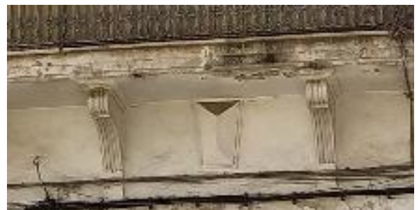
Figure 44 Consoles and decorative keys under the balcony Source: Photographed by author, 2020
