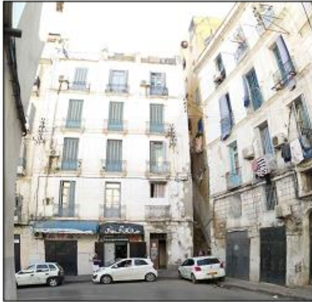
A 5 floors building along Louni Arezki Street Source: Photographed by the author, 2020
