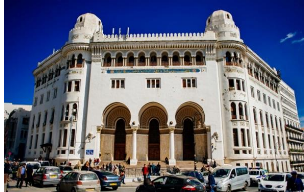
Figure 35 La Grande Poste, Algiers Source : Mahdi Aridj Photography
