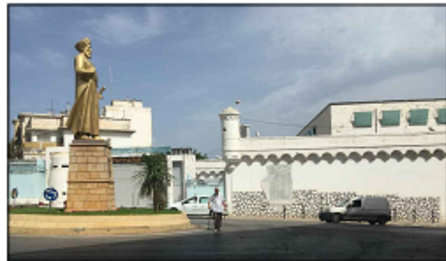
Building to be restored: Serkadji Prison Source: Photographed by the author, 2020
