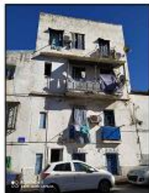
A 4 floors building in a good state along Louni Arezki Street but with no esthetic value Source: Photographed by the author, 2020
