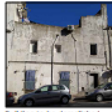
Building to be demolished Source: Photographed by the author, 2020
