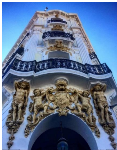
Figure 28 Revenue house, Ernesto Che-Guevara Boulevard Source: twitter
