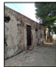
Building to be demolished Source: photographed by the author, 2020
