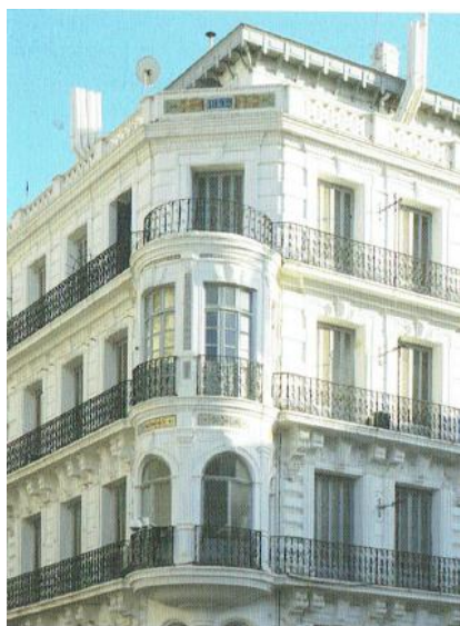
Figure 31 Revenue House ( Old Bégey house) 1892, 37 rue Larbi-Ben-M'hidi Source: PIATON 2016
