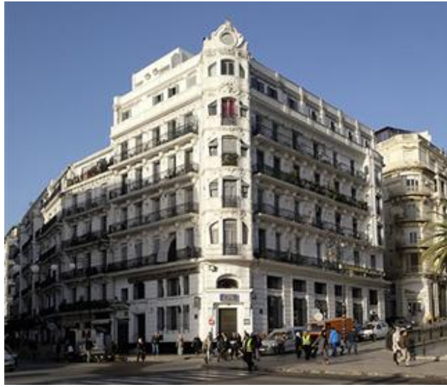
Figure 34 Excelsior hotel - rue Khettabi Alger Source: Google image
