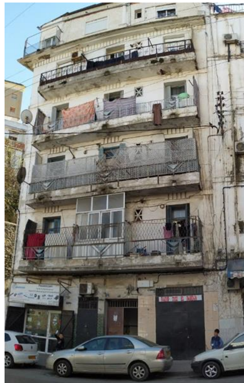
Figure 50 Façade 2, plot 5 Source: photographed by author, 2020
