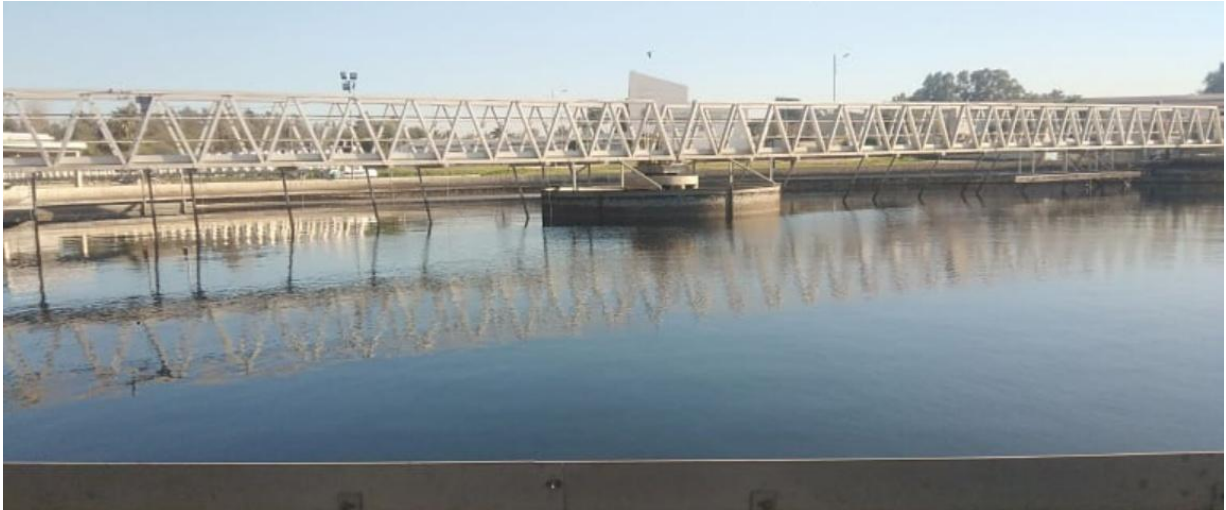
Figure 9 : Clarificateur (photo originale)
