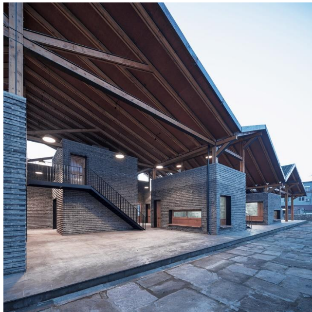
Figure 14: community centre de Hangzhou, (archidaily.com, 2018)
