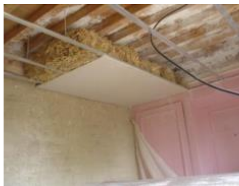
Figure III. 71 le faux plafond
